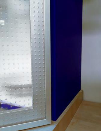
Matching edge banding and 4mm dECOLuxe Solid Acrylic cut to size panels offer a complete cabinet finishing solution.
